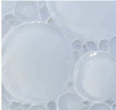
No variations will be seen through the face of the glass tile. In many cases, the mortar's bright white color actually enhances the color of the clear or translucent glass tile.
